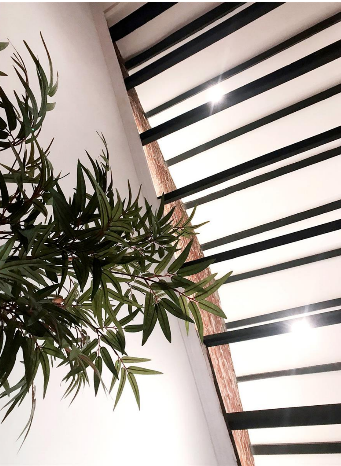
| EXPOSED BRICK WALL W/ FALSE BEAM
