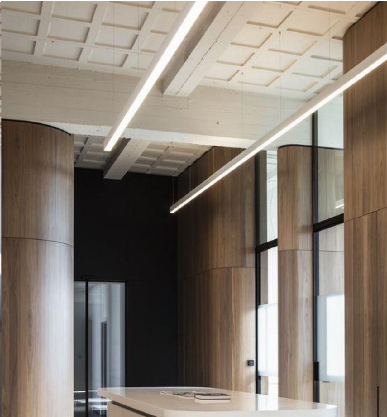
| WHITE COFFERED CEILING BETWEEN BEAMS
